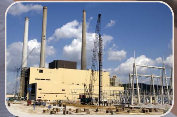
Construction on the new Gilbert Unit
